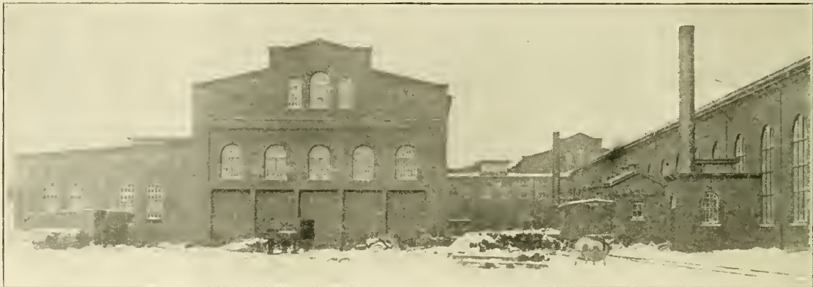
SOUTH END OF BOILER SHOP. FLUE DEPARTMENT LEAN-TO AT THE LEFT. ROLLING SHUTTER DOORS TO FIVE TANK REPAIR TRACKS. BLACKSMITH SHOP AT RIGHT. STOREHOUSE APPEARS AT THE REAR. ALSO SHOWS LAVATORIES AND FURNACE HOUSES AT THE RIGHT.
